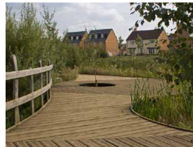
Attractive access to SuDS features can provide multiple benefits.
