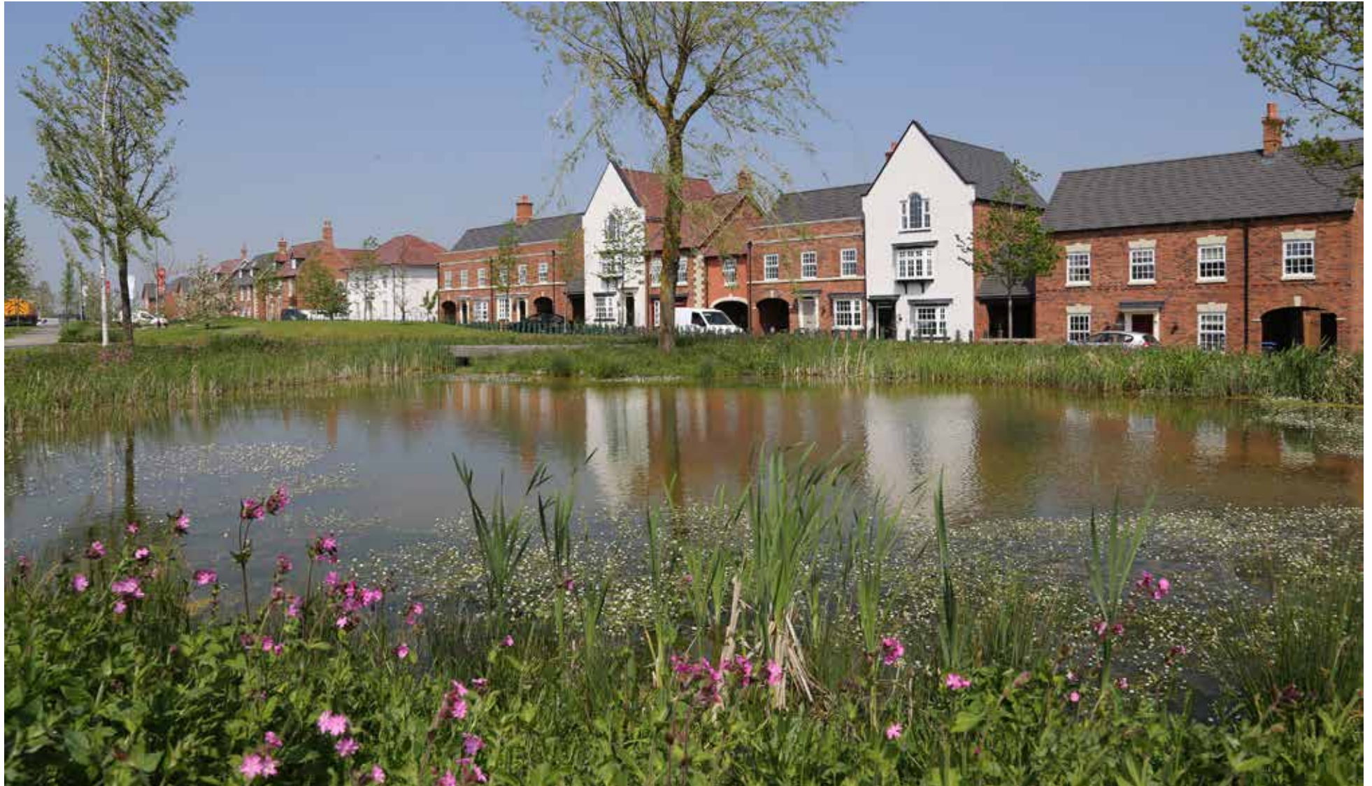
SuDS can add an attractive amenity asset to new residents whilst providing biodiversity benefits
