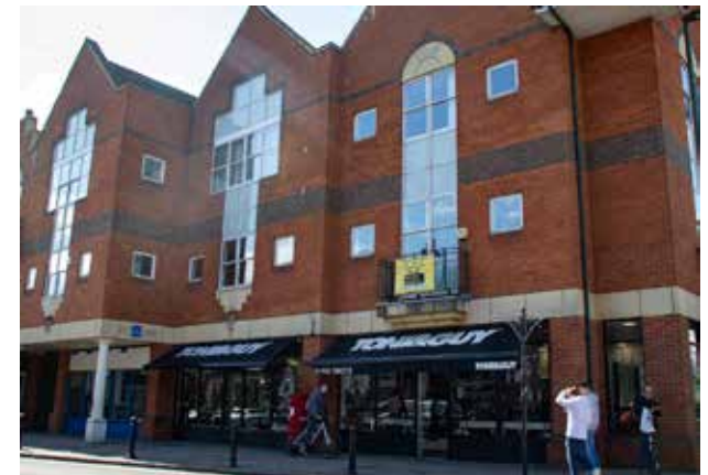
Retail units front onto the pavement providing an active frontage
